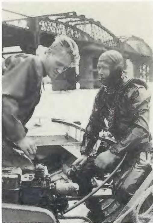
Divers at work surveying the bed of the Mawddach estuary at Barmouth, prior to laying the power cable.
