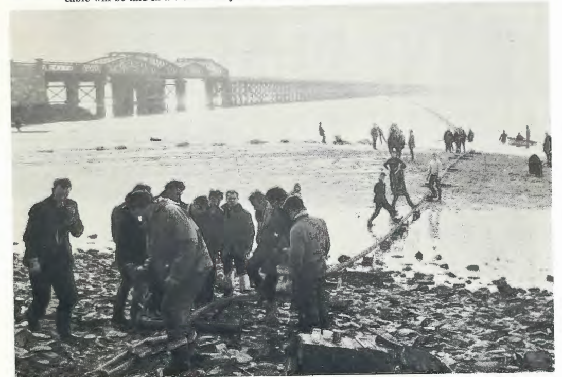
A 20th century sea-serpent straddles the estuary and sprawls across the shore at Barmouth. The shore end of the cable will be laid in a trench and joined to other sections laid underground in the Town.
