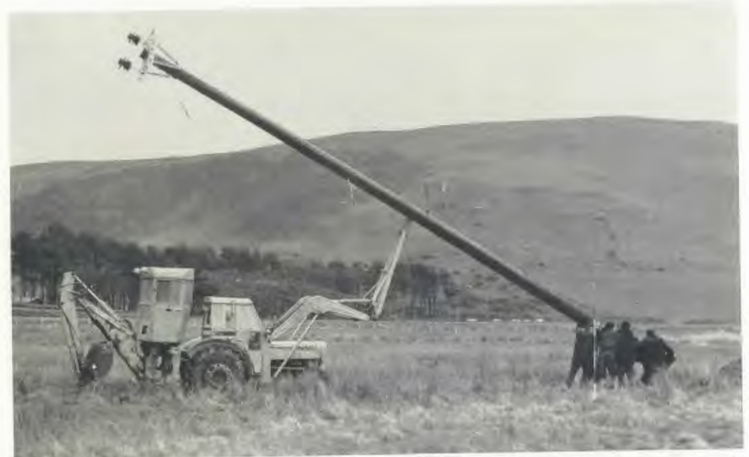
Men and machines co-operate to erect a cable carrying pole on the marshy coastal section north of Barmouth.
